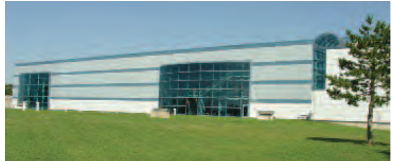
Water Treatment Plant
