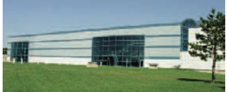
Aurora Water Treatment Facility
