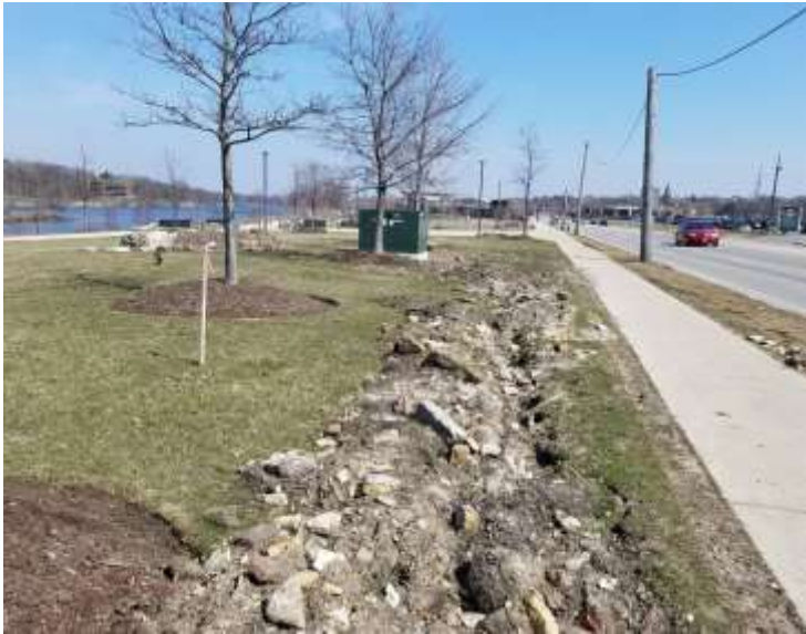
Undergrounding of ComEd Lines, west side of Broadway Ave
