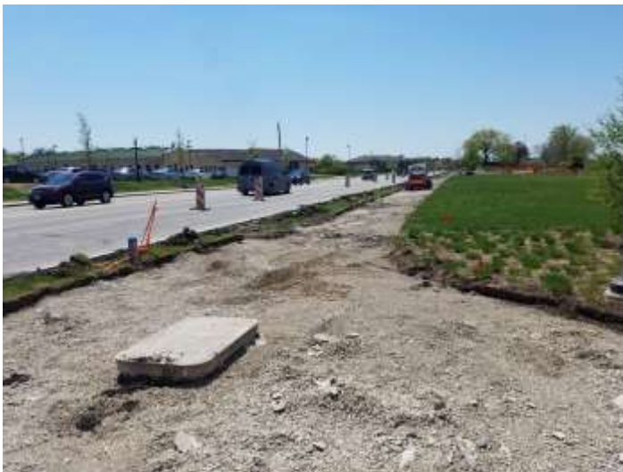
Sidewalk Removal west side of Broadway
