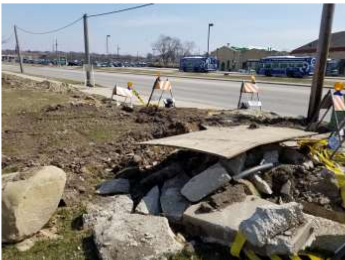
Utility Work (ComEd Relocation)
