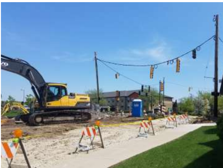
Entrance work at Aurora Township Bldg.
