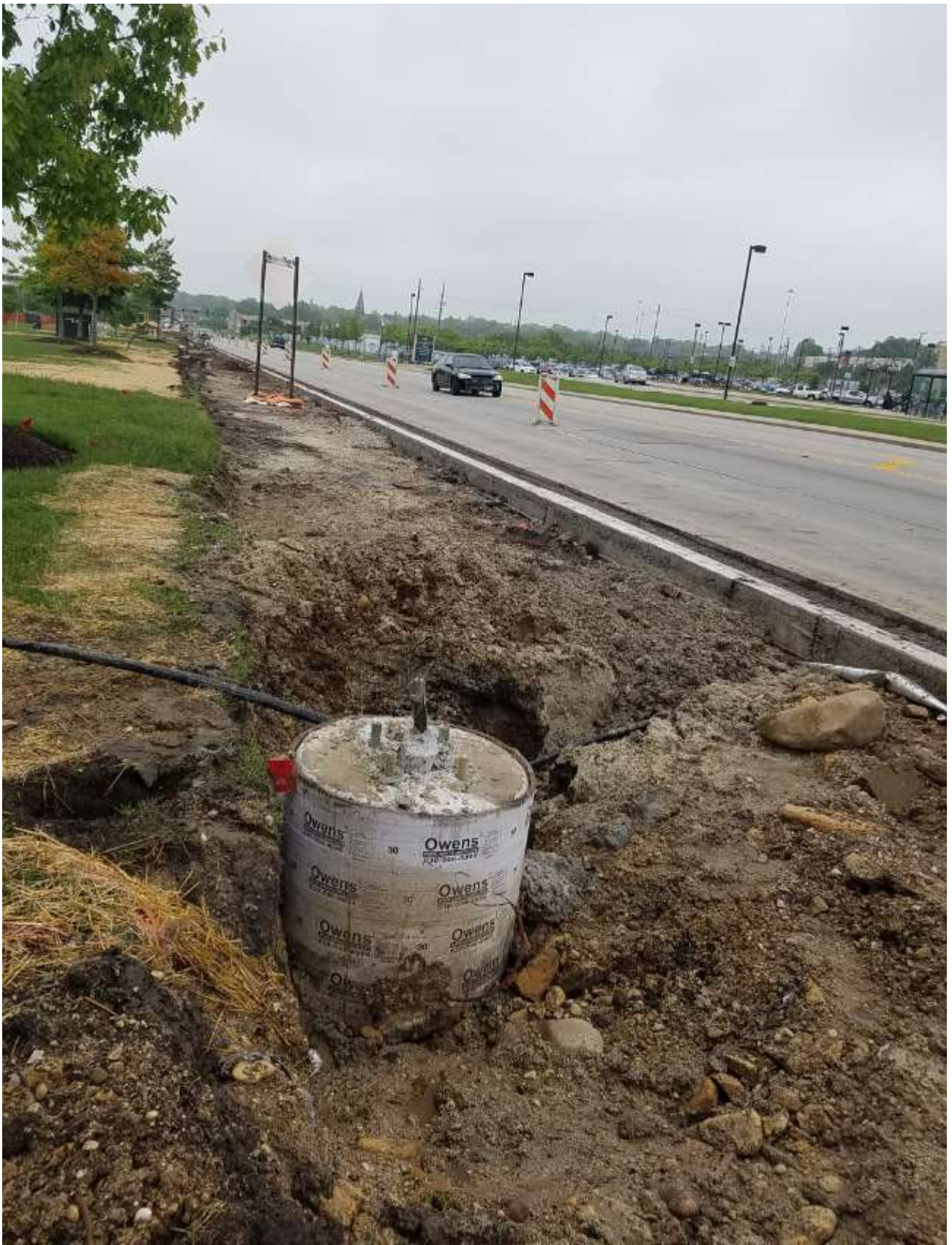
Light pole foundation along west side of Broadway Ave.
