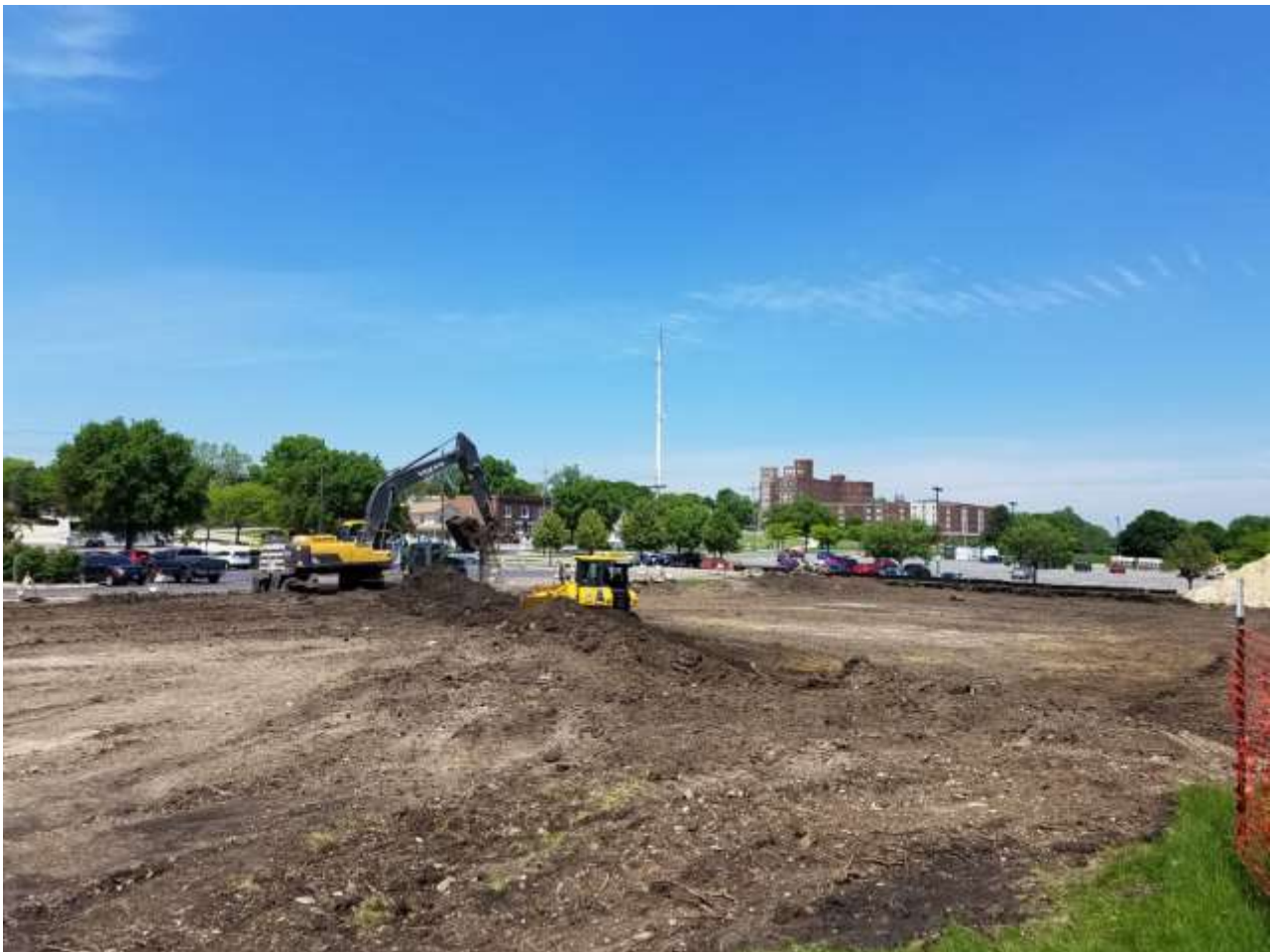
Earth Excavation at Parking Lot X.
