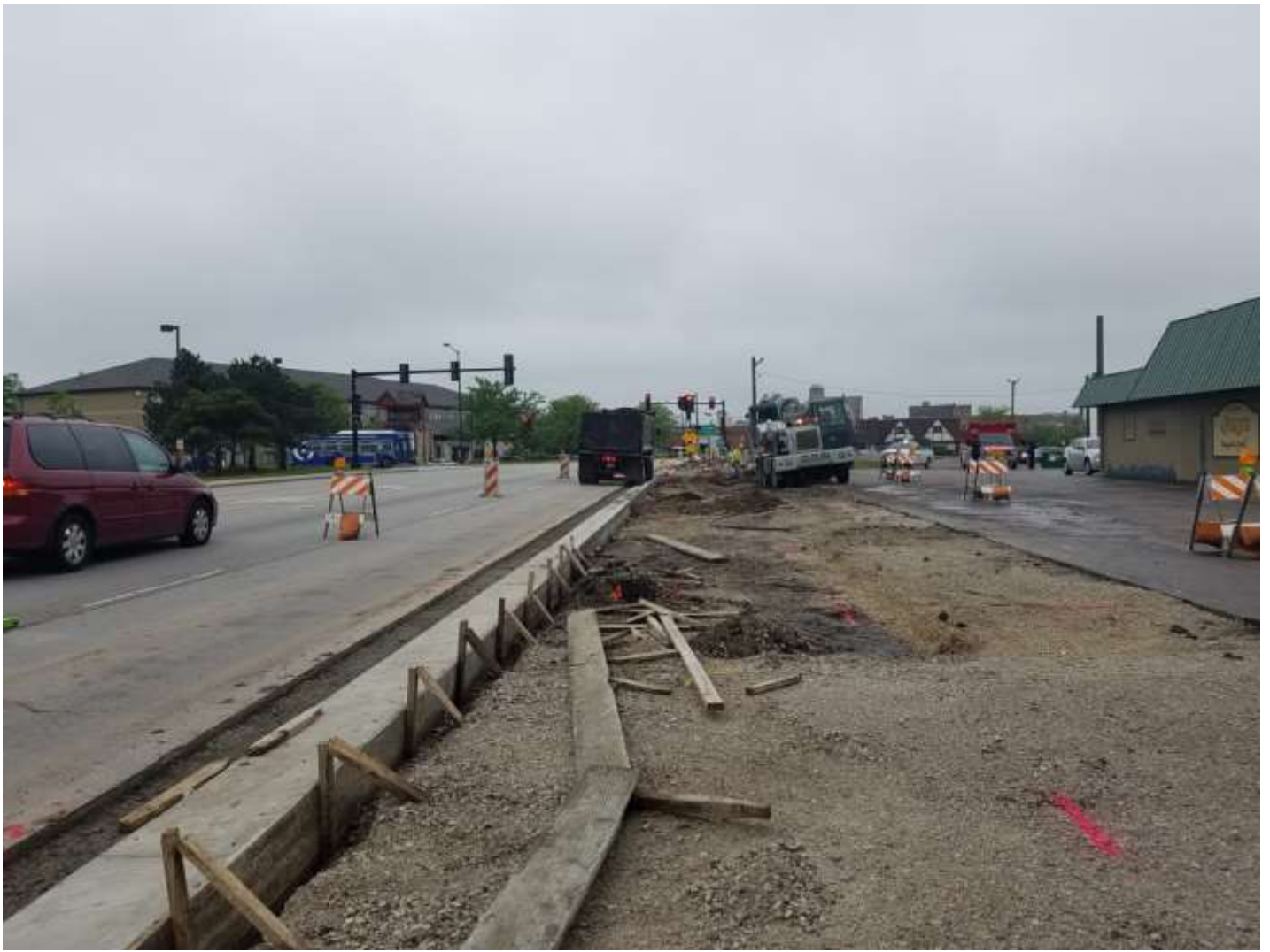
Driveway Prepping at Jakes Bagels.
