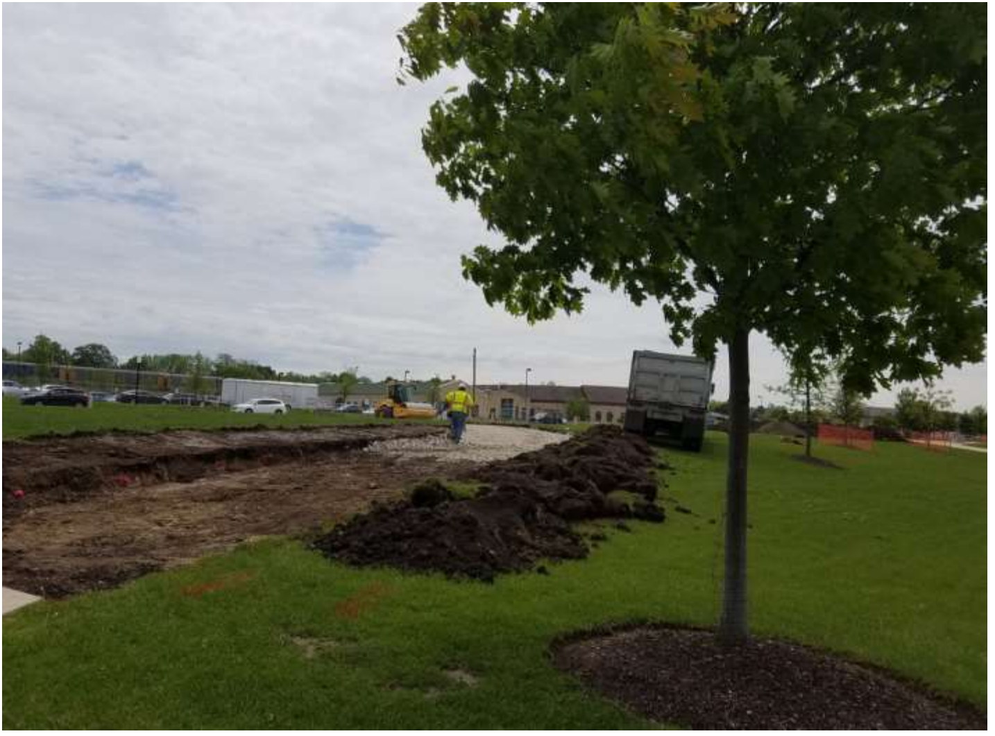
Earth Excavation of Construction/REP access road.
