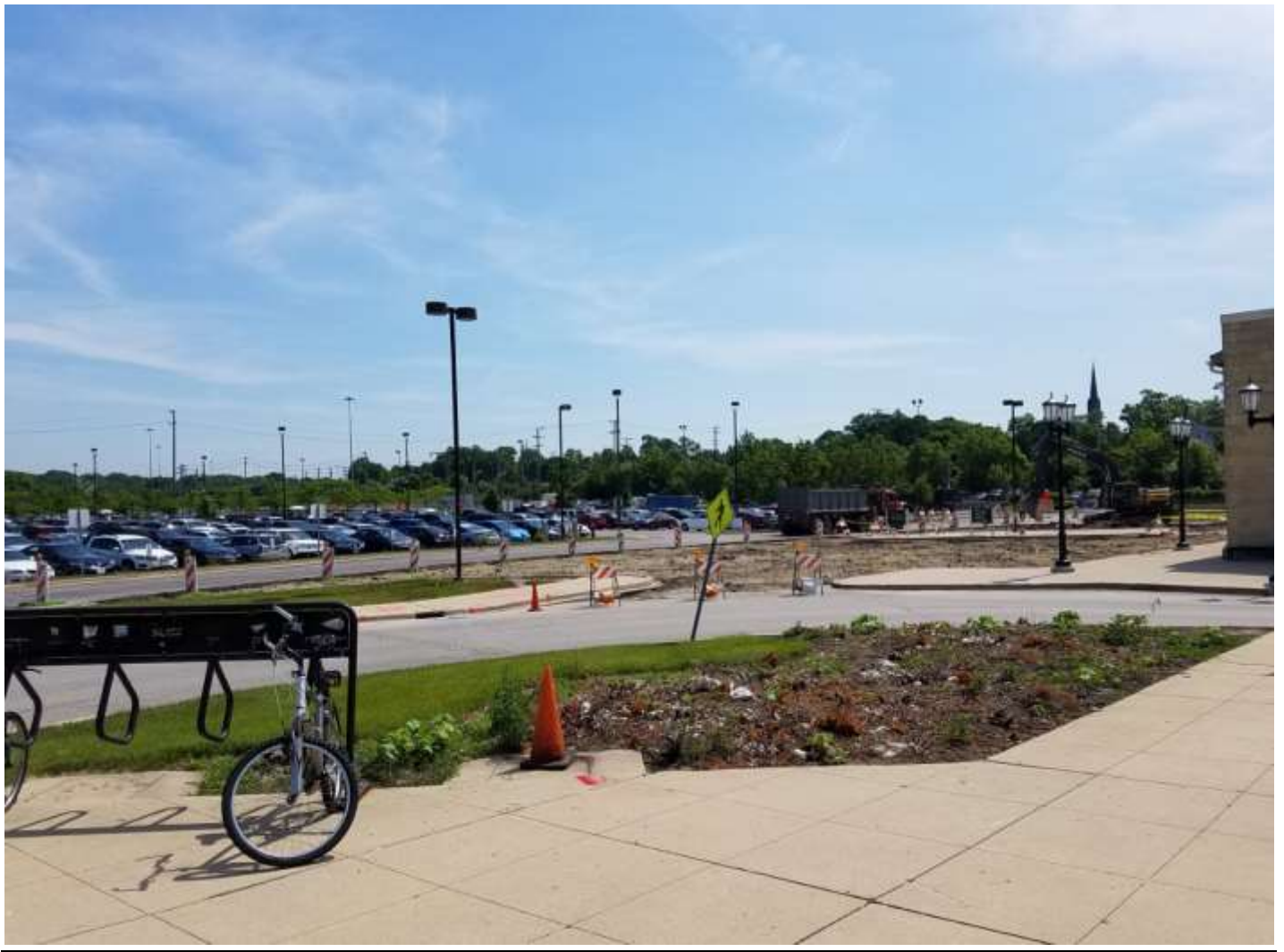
Stage 2 Work- Pavement Removal, north of ATC Building 06/07/2018
