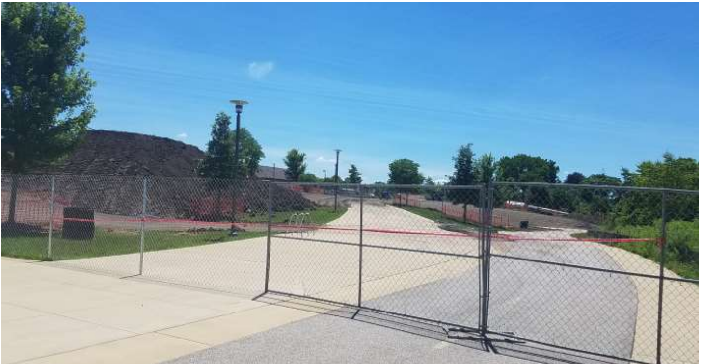
Stage 2. Construction fencing and prep area for causeway construction. Looking SW from RiverEdge Park sidewalk.
