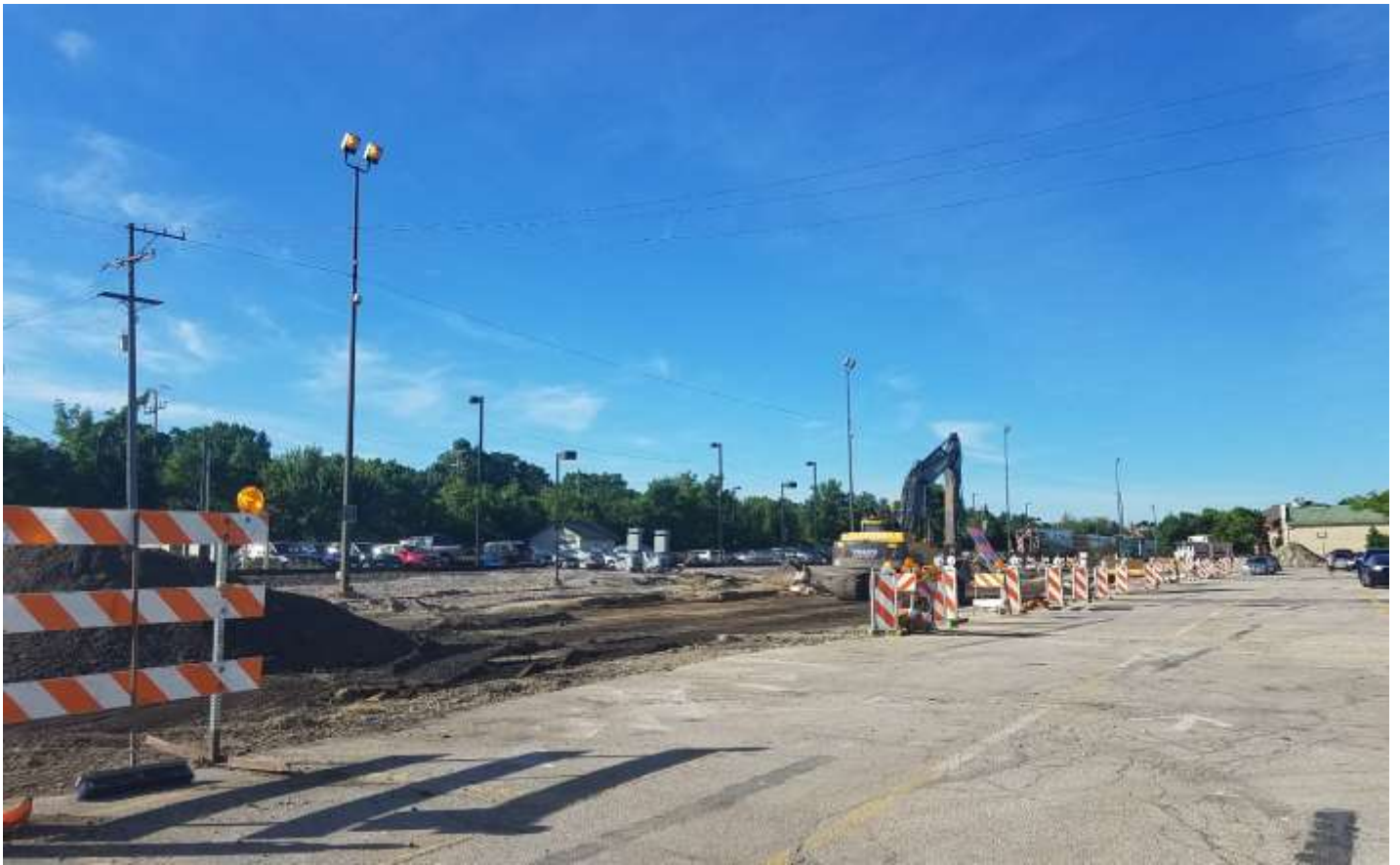
Stage 2- Earth Excavation along west side of R.R Track. Looking SW
