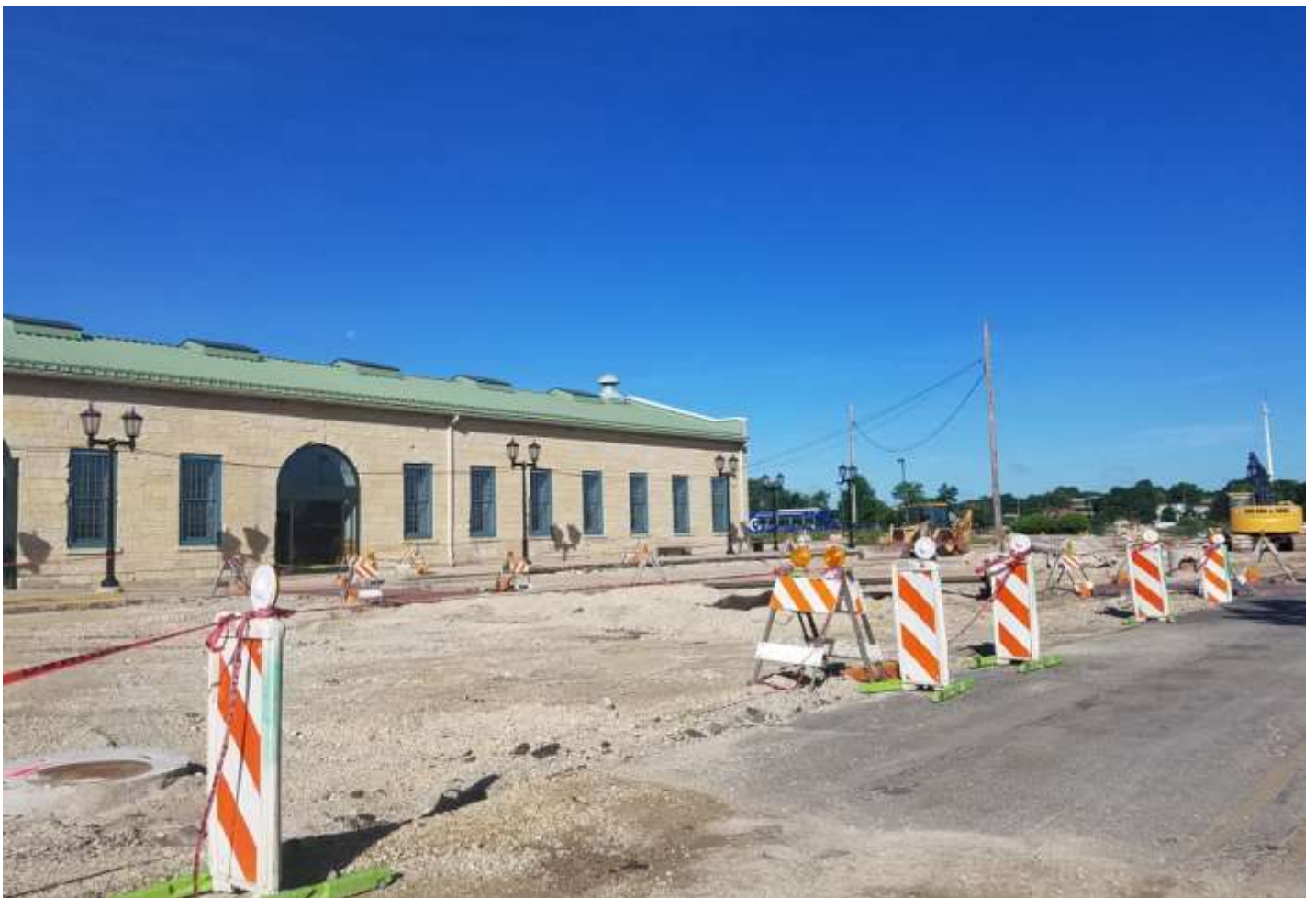
Stage 2-Earth excavation along north side of ATC Bldg. Looking SW.
