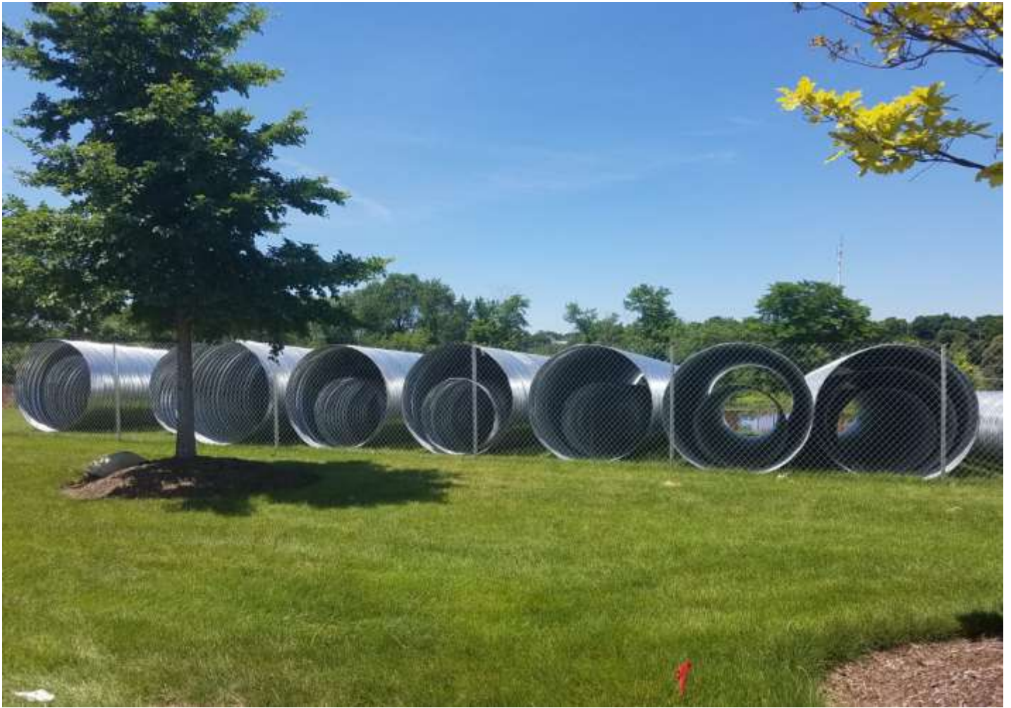
Stage 2- Culverts staging for causeway construction. East side.
