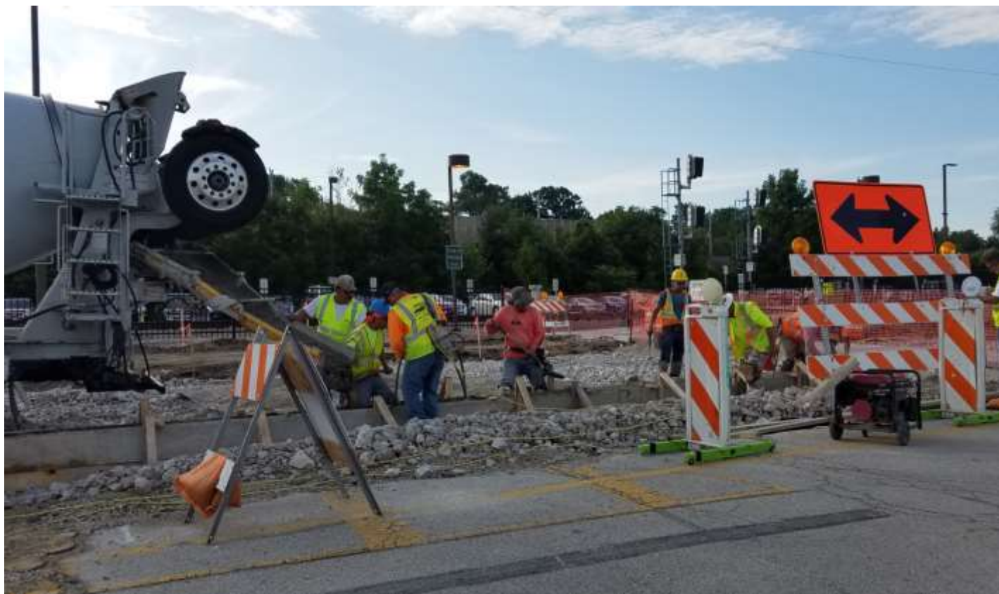
ATC Parking Lot- Pouring curb and gutter.
