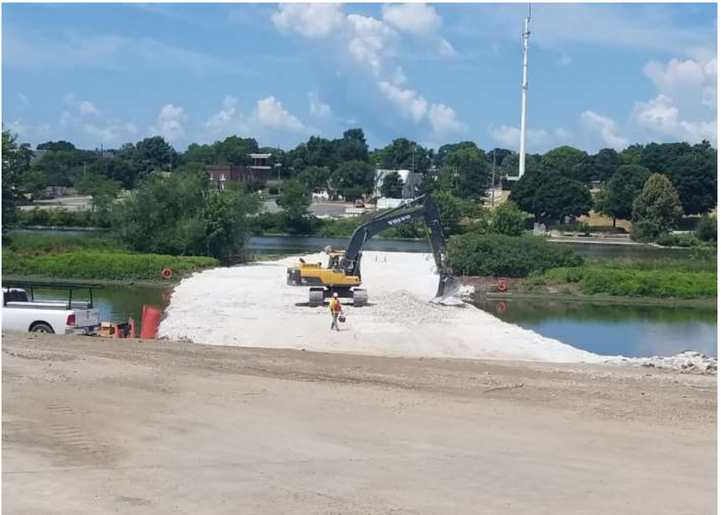
Stage 2. Causeway Construction Continue. Looking West
