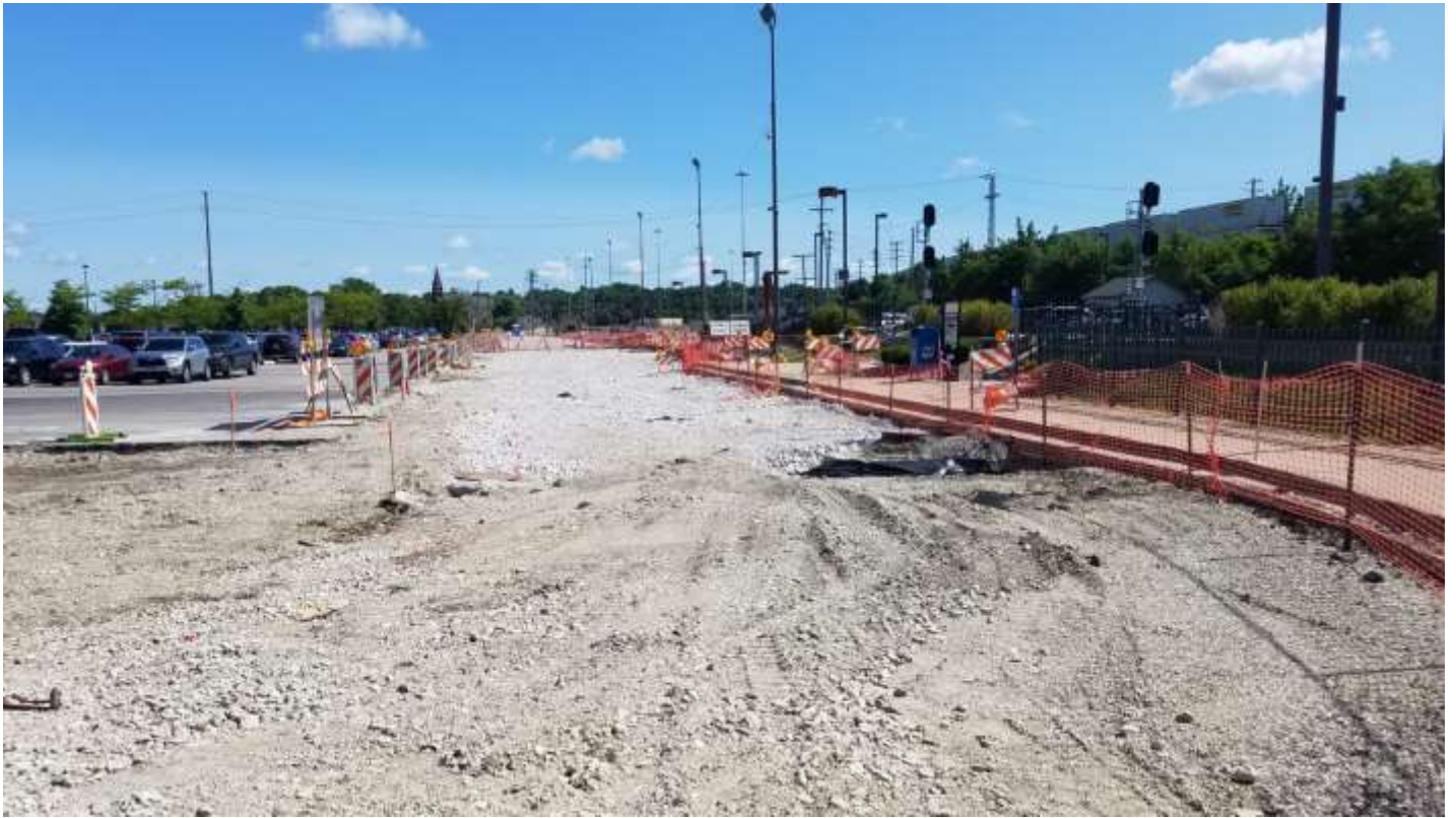
Stage 2- ATC Parking-Pace Staging Area- Continue earth excavation.
