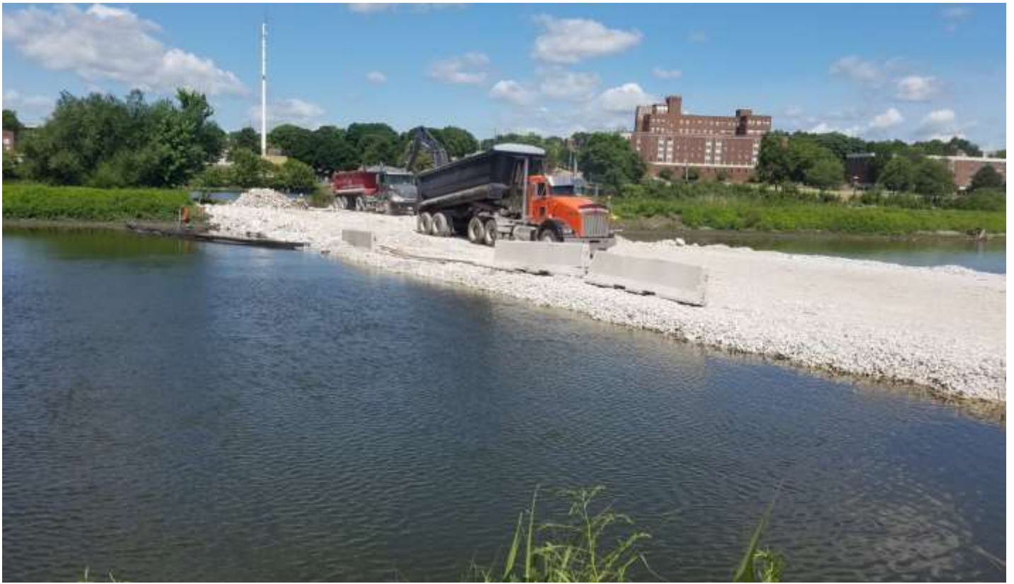
Stage 2- Causeway Construction continue. In stream work. Looking west.
