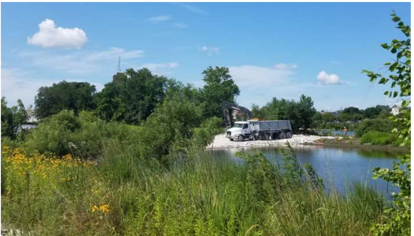
Stage 2. Causeway Construction (in stream work). Looking SW.
