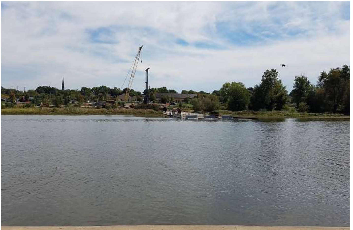
Drilling for pier # 6-looking east across Fox River.
