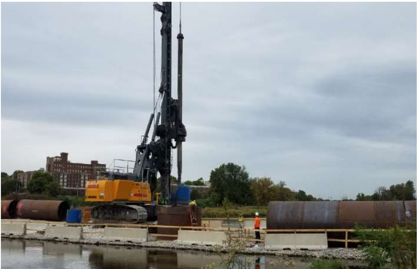
Drilling of Pier # 6-
