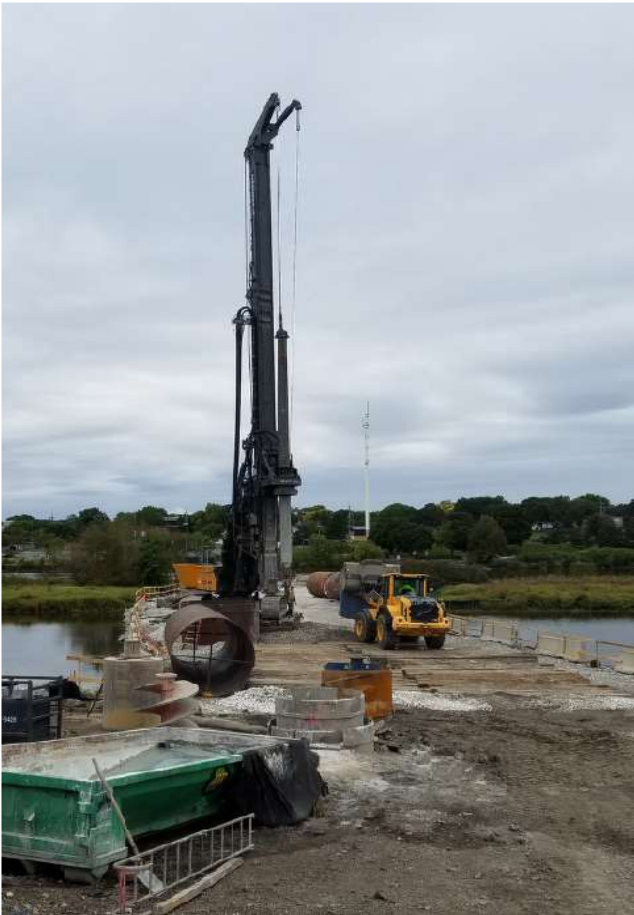
Drilling of Pier # 6-
