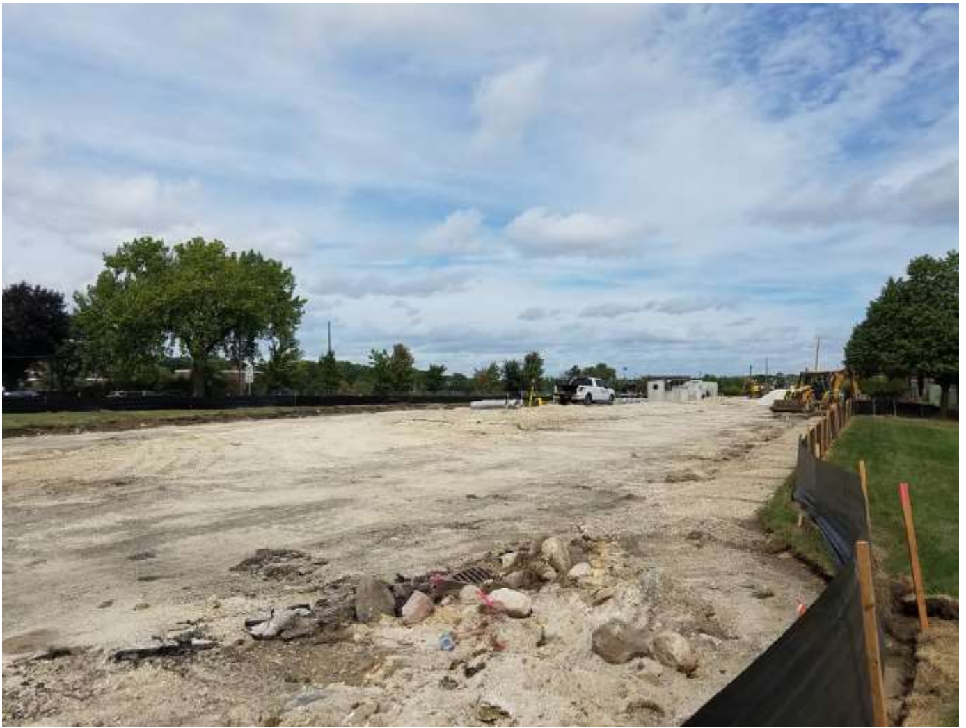
Stage 3 construction-paving removal and rough grading.
