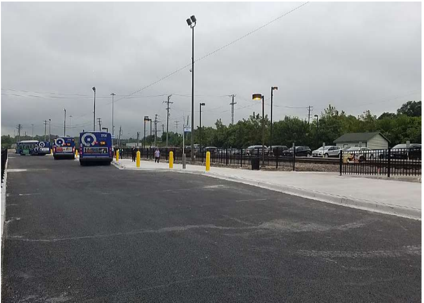
ATC Parking/Pace Staging Area- Completed Pace Staging Area looking north. Open to commuters.
