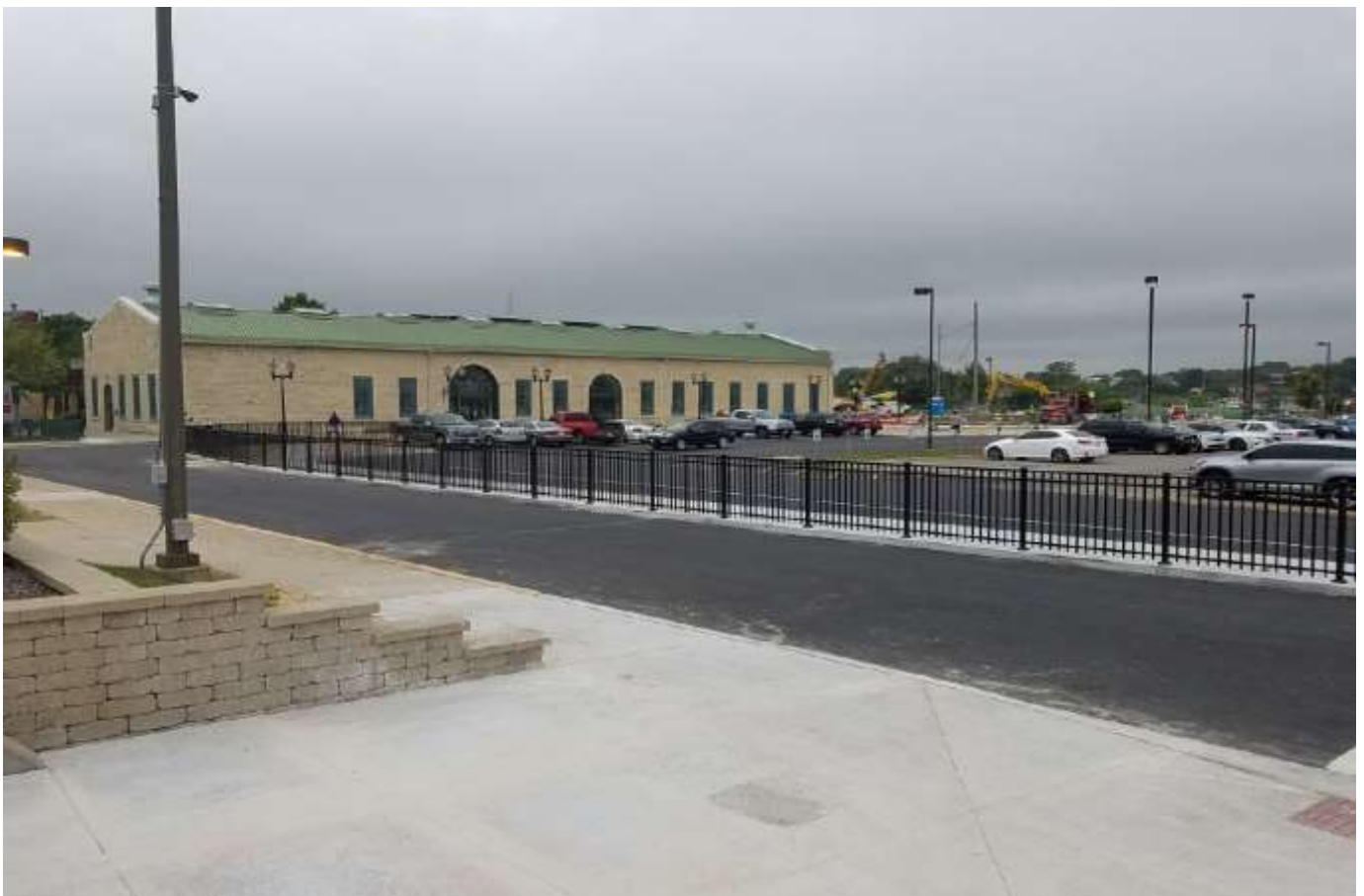
ATC Parking/Pace Staging Area-Completed Area
