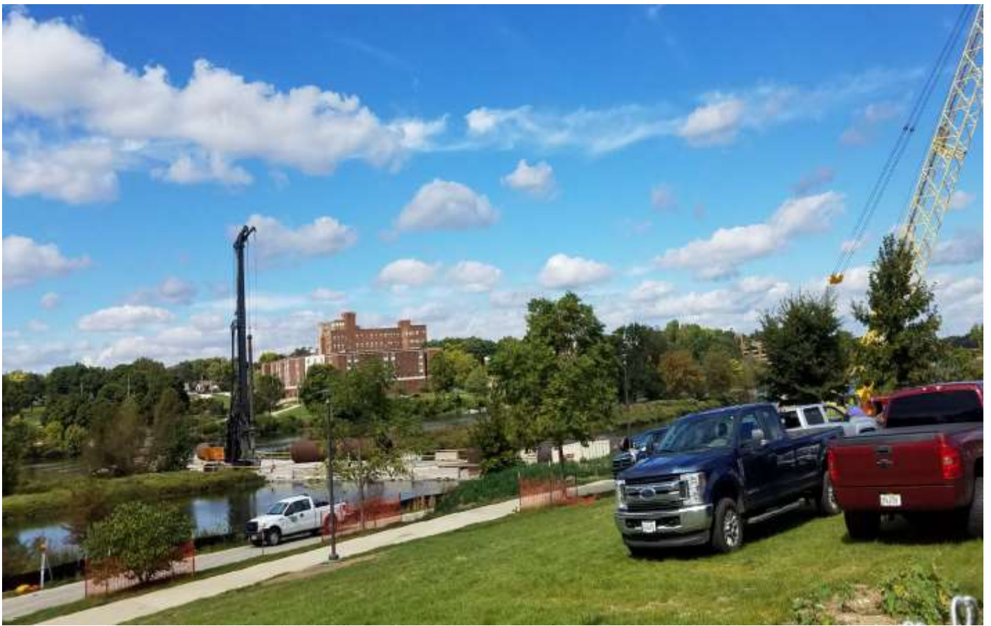
Contractor staging for drill shaft-looking west
