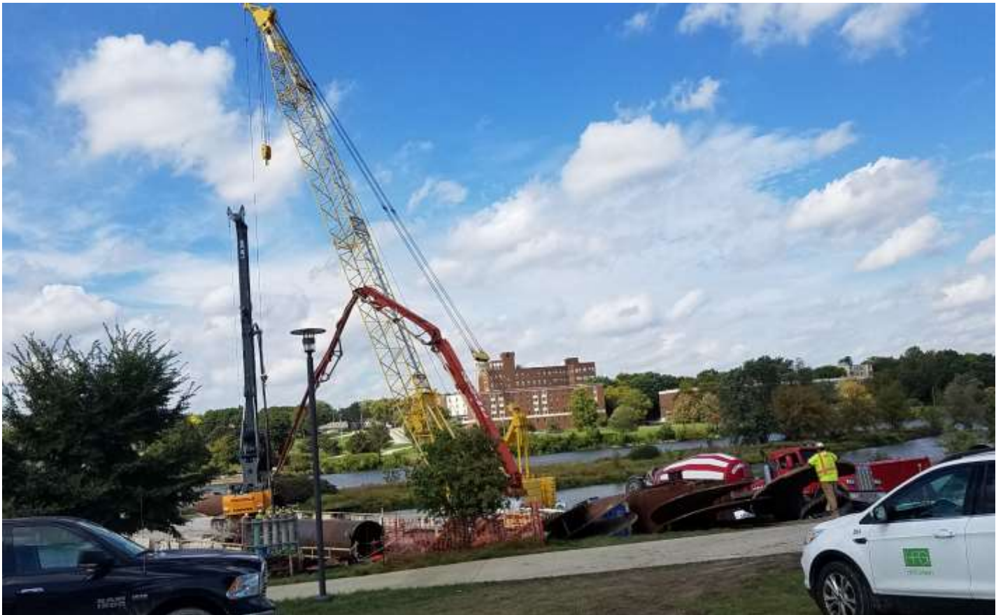
Pouring of concrete at Pier # 6
