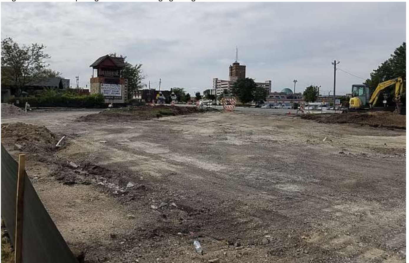
Broadway Ave Entrance- looing south.
