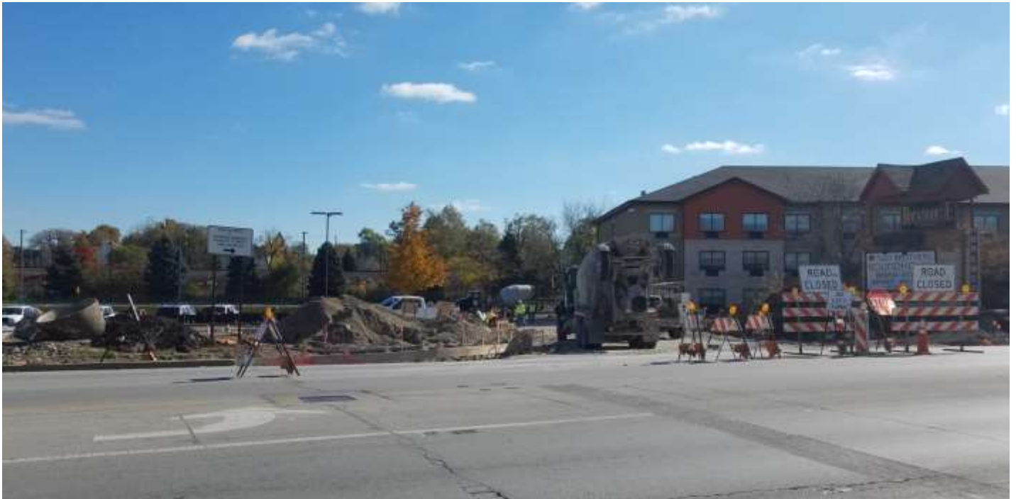
ATC Parking Lot/Pace Staging Area- Pouring curb and gutter. 10/28/2018
