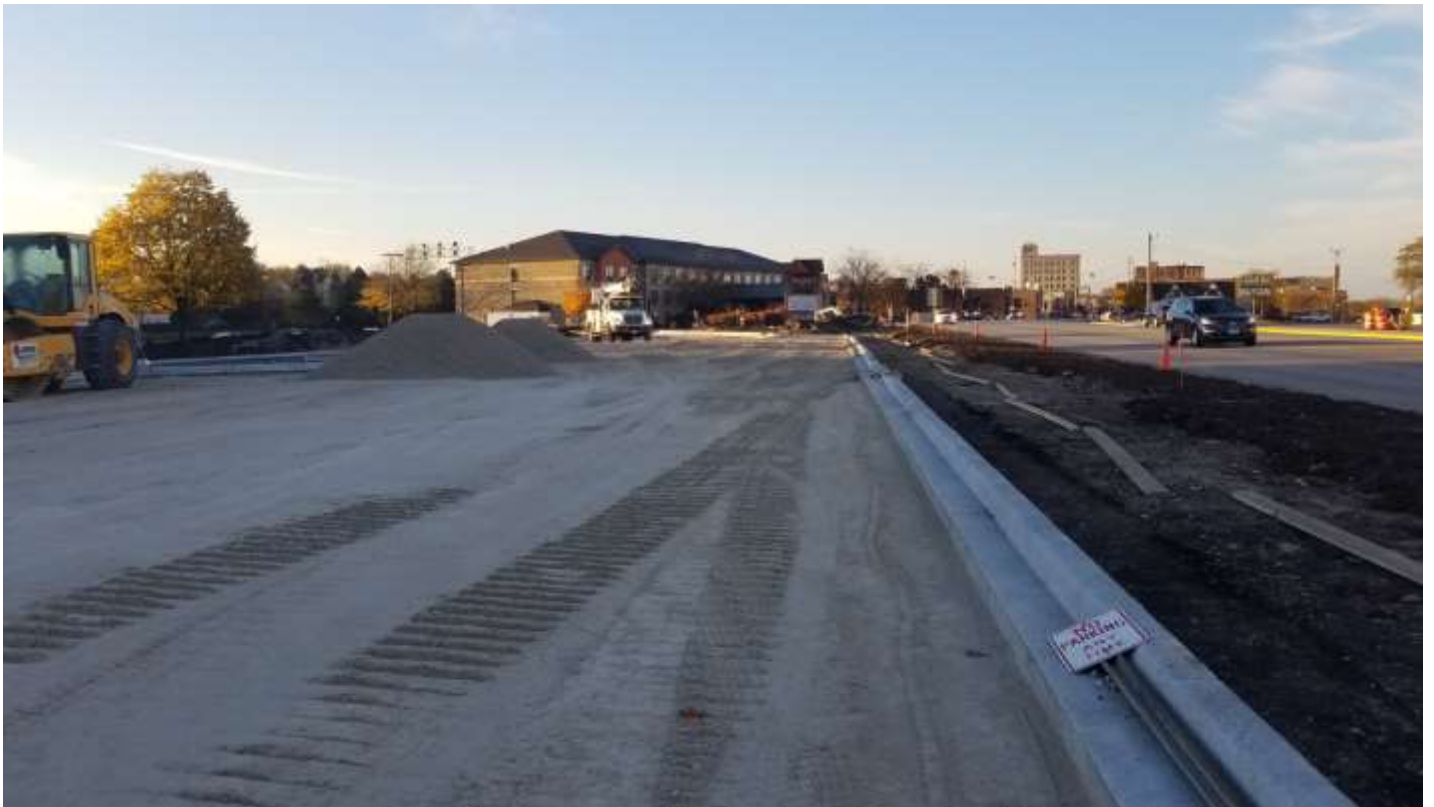
ATC Parking Lot/Pace Staging Area- Looking south. Placing of capping aggregates. 11/02/2018
