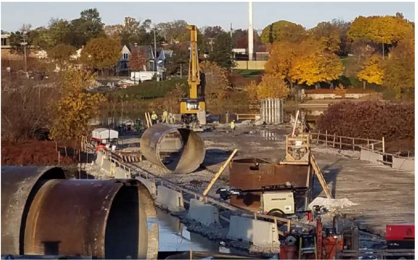
Drilling Shaft at pier # 3 -looking west 11/02/2018
