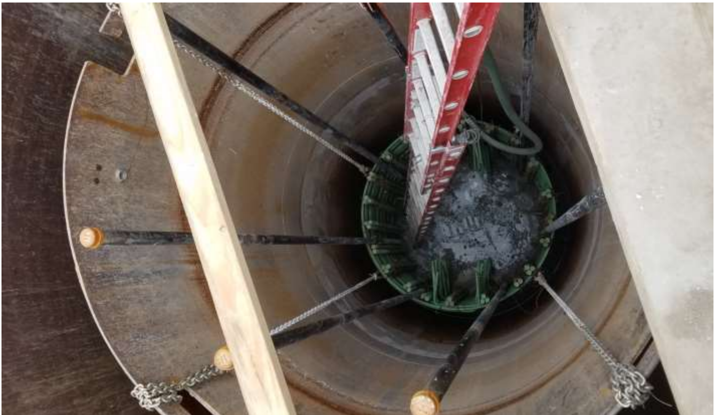
Inside Pier # 6- after concrete pour and installation of reinforcement steel cage.
