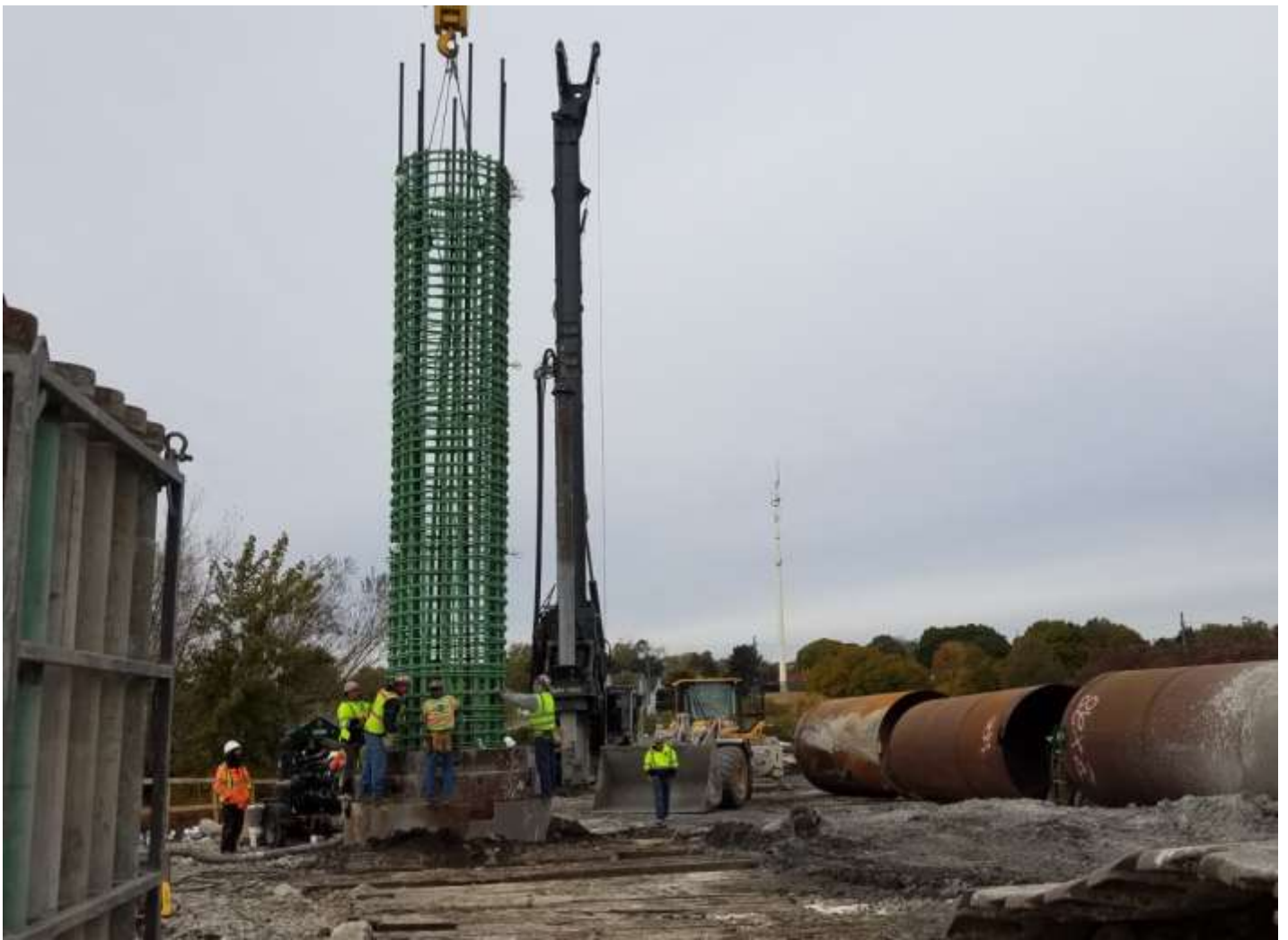
Lowering of reinforcement steel cage at Pier # 5. 10/25/2018
