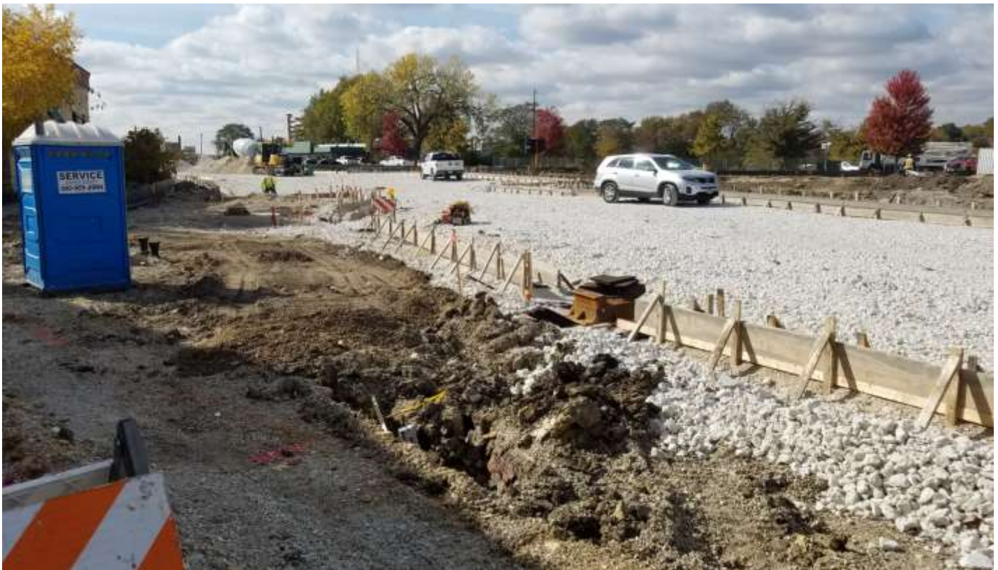
ATC Parking Lot/Pace Staging Area- 10/24/2018
