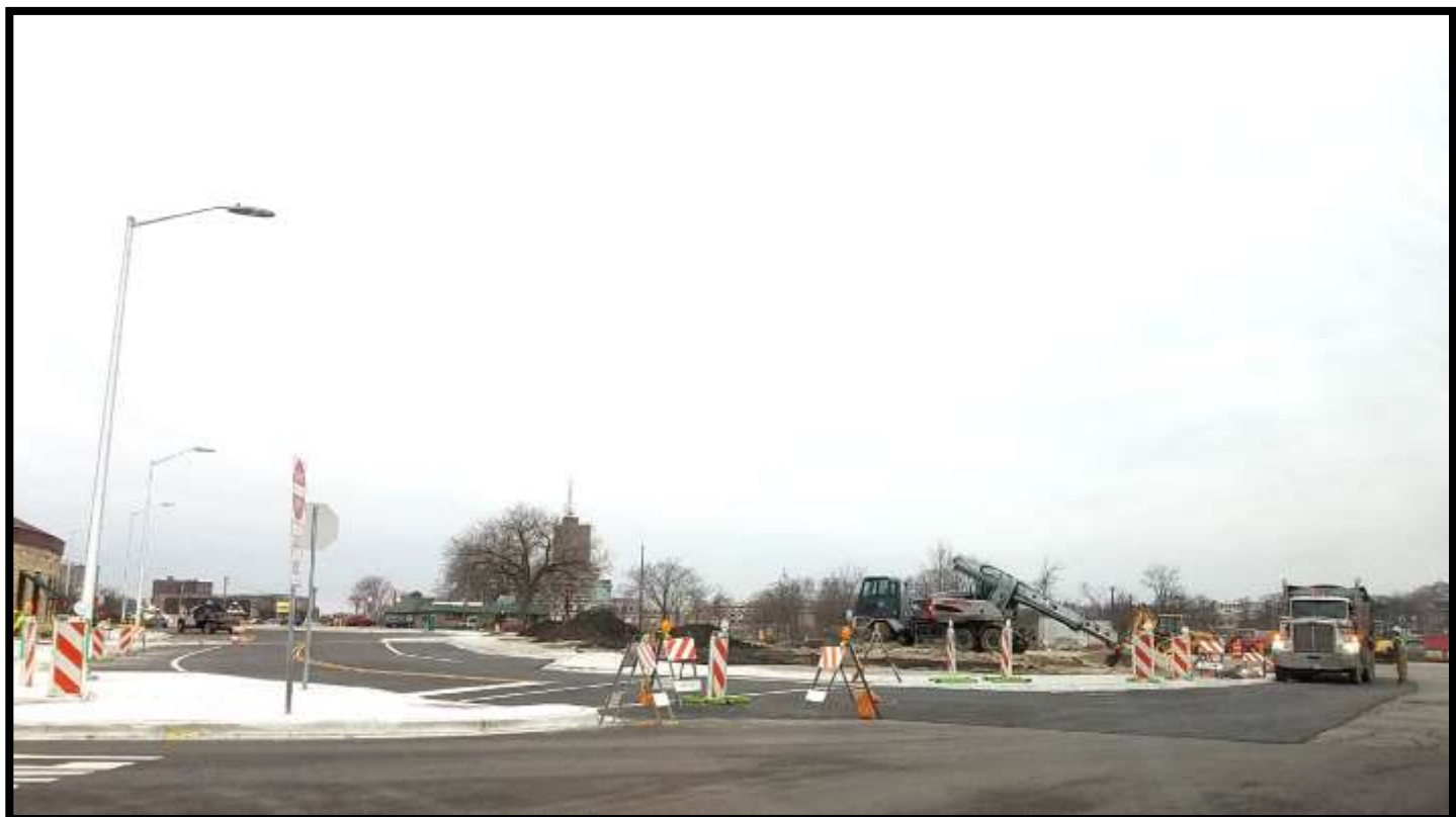
ATC Parking Lot/Pace Staging Area- Looking north. Placing topsoil and backfilling behind sidewalk 12/06/2018
