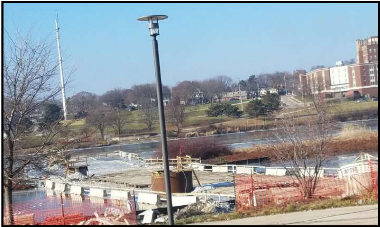
Piers Construction- looking west . 12/10/2018
