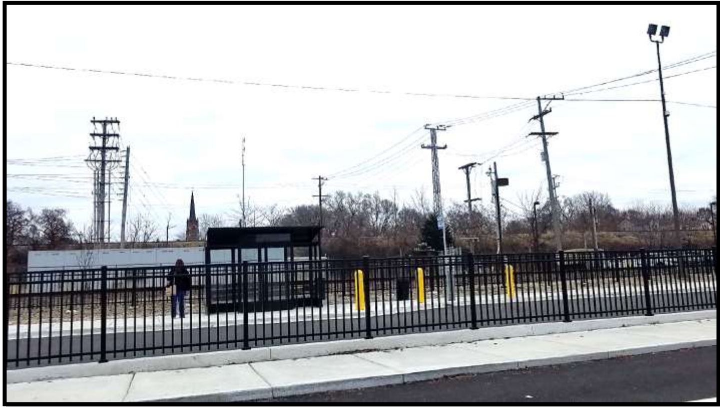
Installed Pace Shelter- Pace continues shelters installation. 12/10/2018
