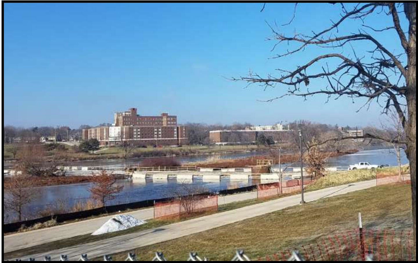
Piers Construction- looking NW. 12/10/2018
